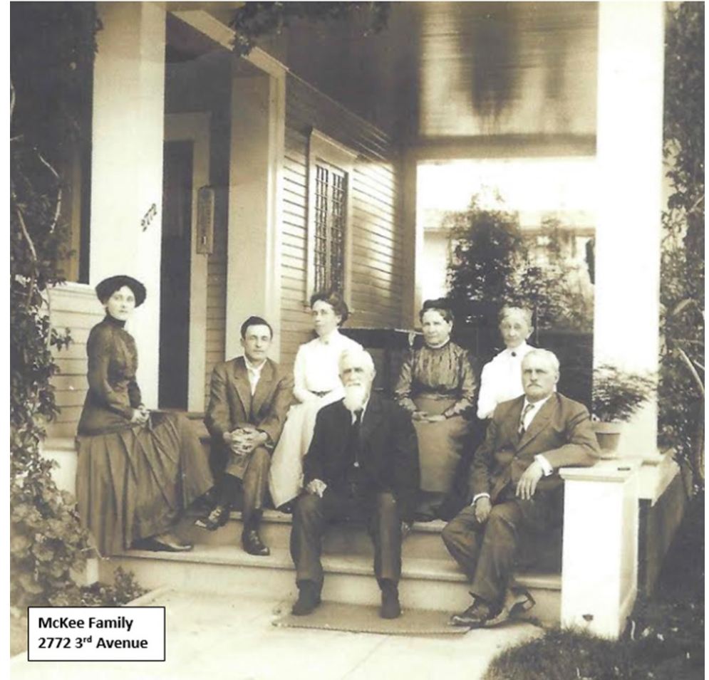
L.D. McKee Residence 2772 3 rd Avenue Early 1900s
